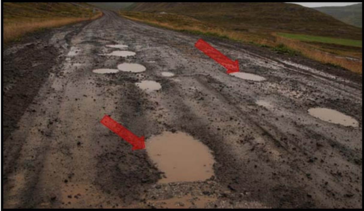
**Figure 3: Typical pothole pattern during wet conditions.**
